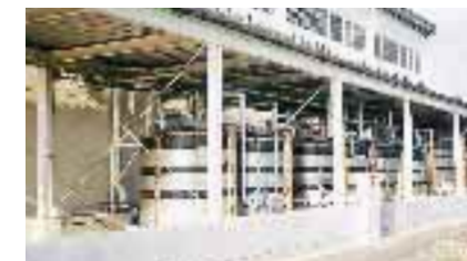
Concrete walls surrounding liquid waste tanks
