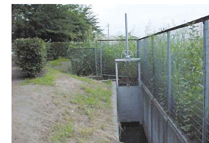
Installation of watergates to adjoining public water systems
