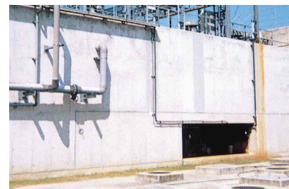
Wastewater treatment facility/underground leakage inspection pit
