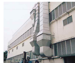
Noise reduction duct installation (Kashiwa plant)
