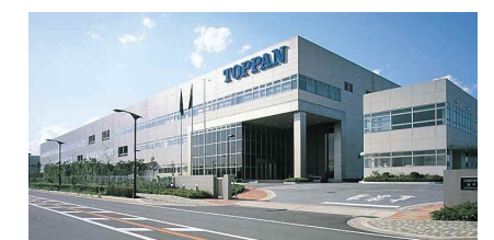
Sakado plant (Information & Networks)
