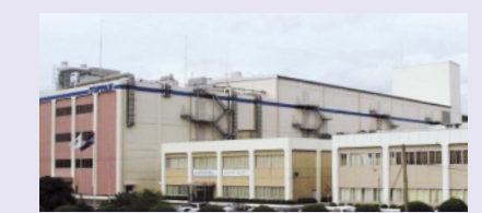
Electronics Division, Kumamoto plant (Production plant in the Electronics field)
