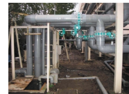
Installations of emergency shut-off valves on the final drainage line
