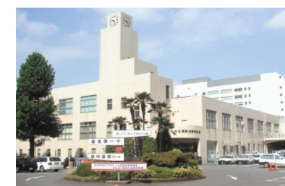
Itabashi plant (Information & Networks)
