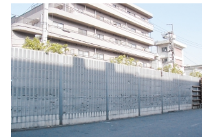
Soundproof wall installation (Toppan Seihon Co., Ltd.)
