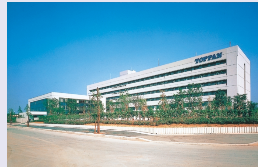
Toppan Technical Research Institute
