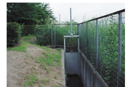
Installation of watergates to adjoining public water systems
