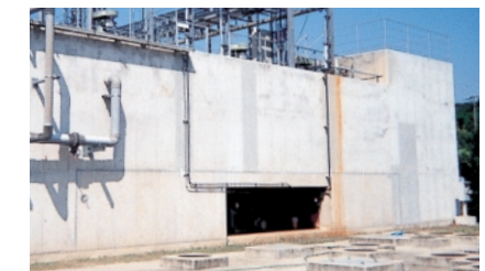
Wastewater treatment facility/underground leakage inspection pit
