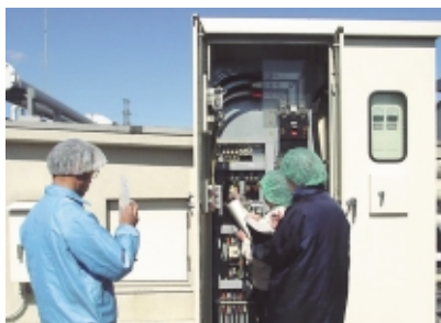
Energy saving inspection at site
