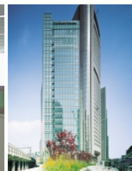
The Shiodome building
