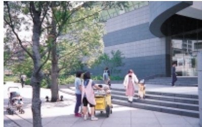
Space open to the public nearby the Toppan Koishikawa Building
