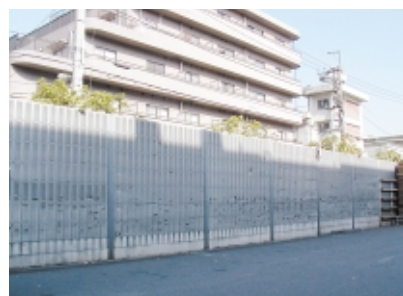
Soundproof wall installation (Toppan Seihon Co., Ltd.)
