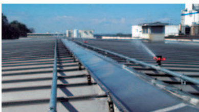
By placing and sprinkling water onto the tops of factory roofs, radiant heat from the sun's rays in summer is reduced, decreasing the burden on air conditioning. (Kumamoto plant)
