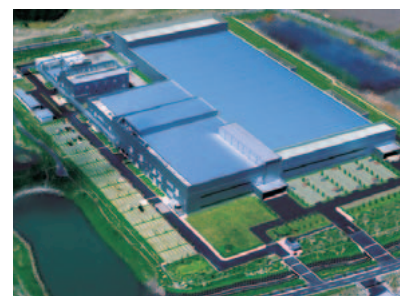
The Mie Plant (Kameyama City, Mie Prefecture: Plan showing the plant following completion of the current expansion work.)
