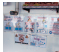
The Company renews its underground effluent tanks, and increases the use of warning devices against the possibility of emergency situations including leakages.
