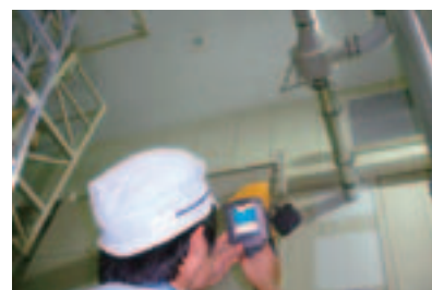
Inspecting heat release spots by thermography
