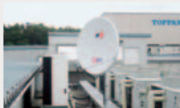
Parabola antenna to receive radio signals of Earthquake Early Warnings
