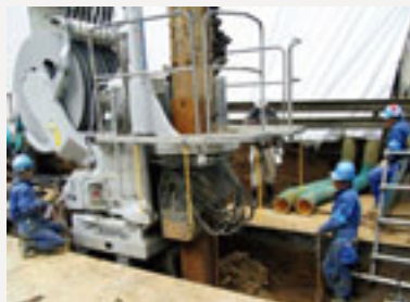
Extension work of the water-shielding wall
