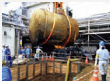
Removal of the underground tank
