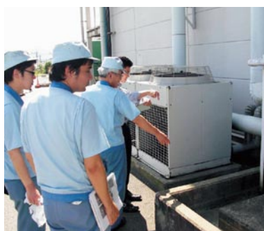
Internal environmental audit inspection
