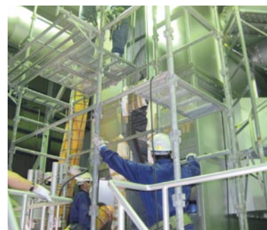
Replacement of effluent-gas treatment equipment
