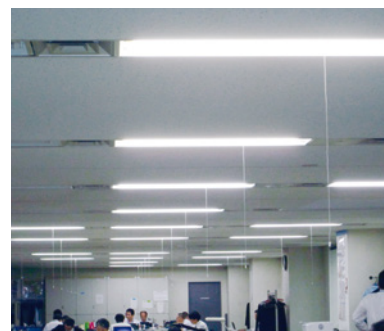
All fluorescent lights at the head office replaced with LED lights
