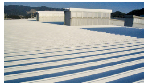
Roof coated with heat-shield painting (Fukuoka Plant)
