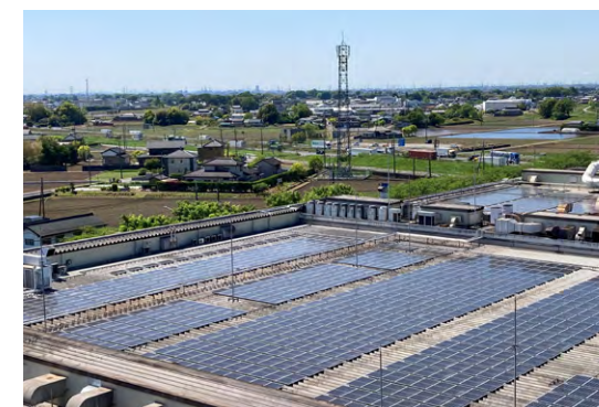
Roof of B building, Satte Plant of Toppan Decor Products
