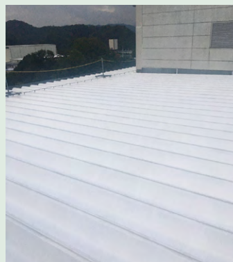
Segmented roof with a thermal barrier coating
